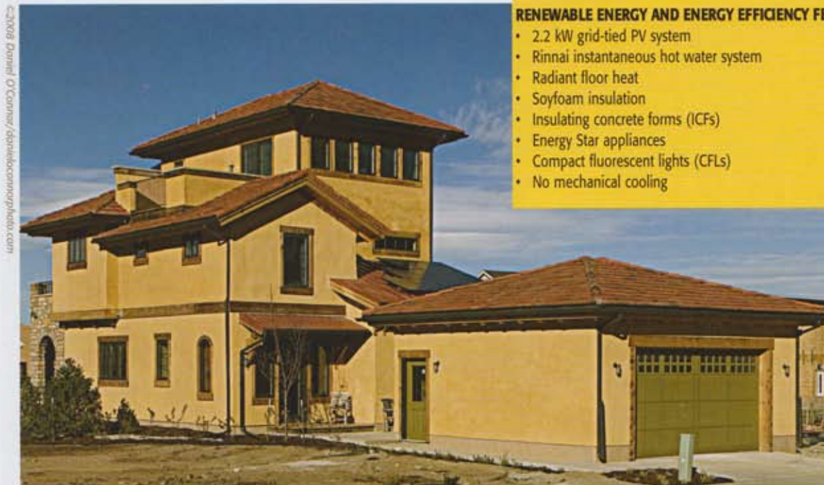
Merten Homes' new straw bale home in Old Town North in Fort Collins boasts R-28 walls, R-72 ceilings, and a 2.2-kilowatt grid-tied solar electric (photovoltaic or PV) system.
